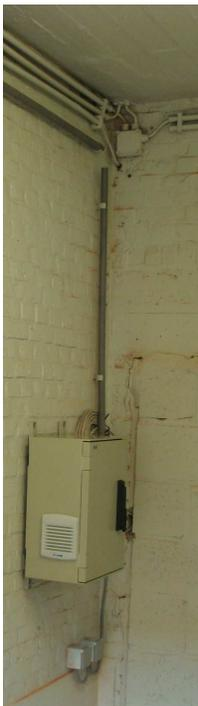
An industrial enclosure that contains the data acquisition module and an industrial computing unit. The box is installed in the vicinity of the track up to a distance of 150 m.
